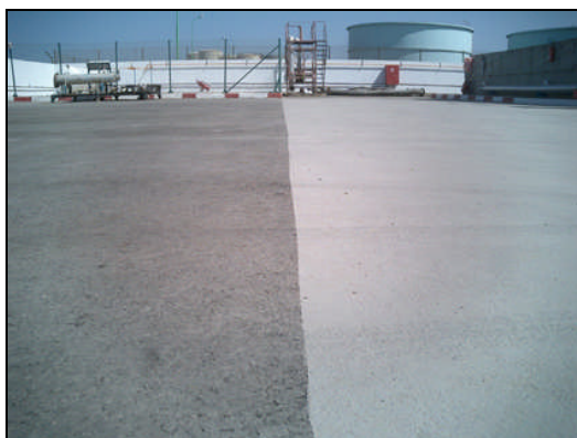
Bitumen and Fuel storage area
