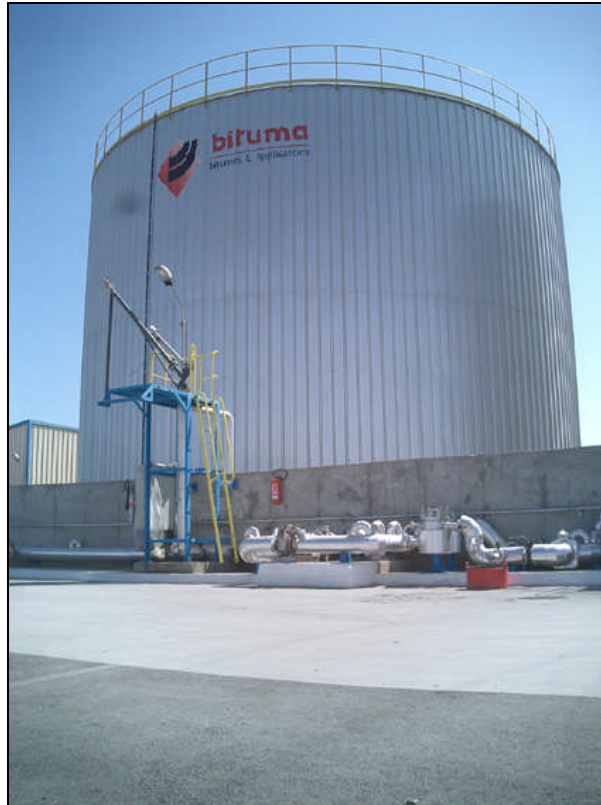
Bitumen and Fuel storage area
