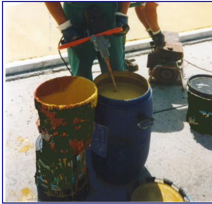
Homogenizing before application
