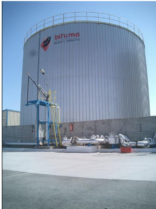
Bitumen and Fuel storage area
